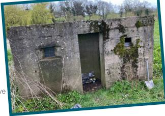
formwork. Concrete was mixed and poured over several days as the pillbox grew, creating a bulletproof bunker from which soldiers could defend the crossing points of the three rivers.
