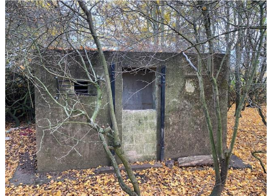
Figure 5. This pillbox conversion on the Burton Washlands has the bottom section of the entrance blocked up. The gate has been torn off by vandals.
