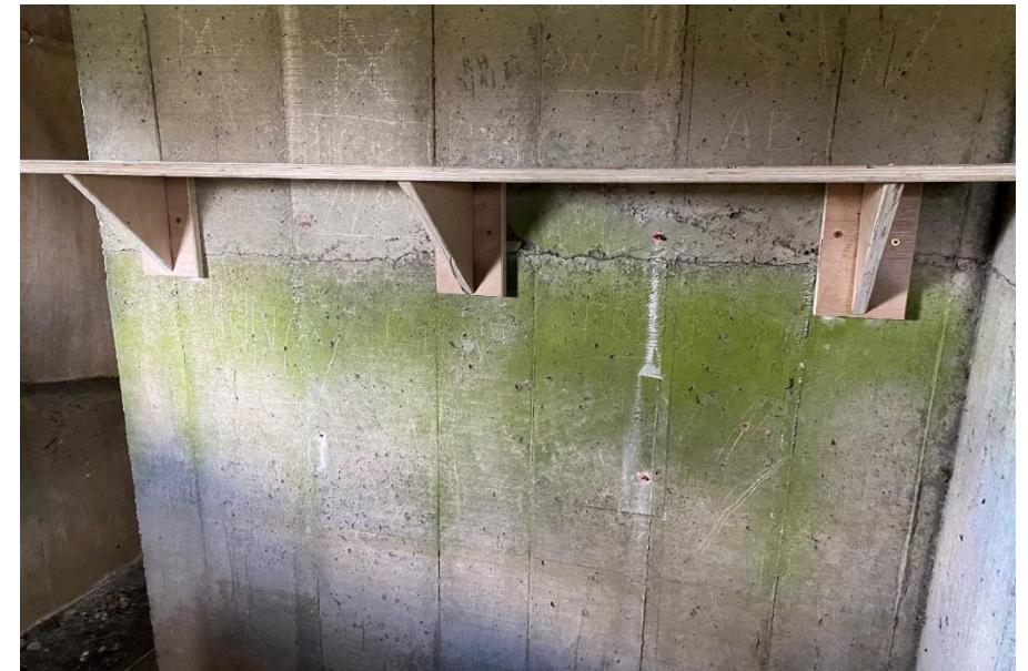
Figure 7. A plywood nesting shelf fitted to either side of the internal blast wall.
