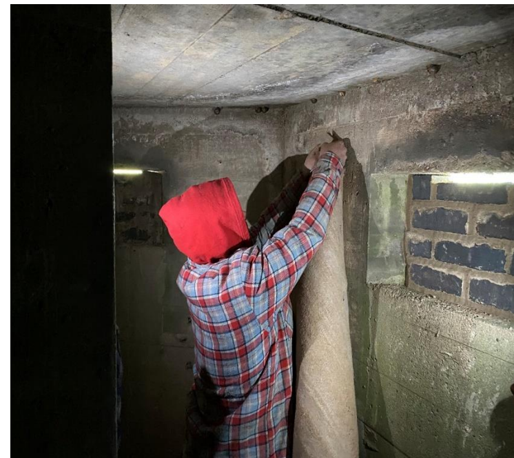
Figure 9. Hanging hessian for bat use. Note also the ~30mm 'letterbox' gap in the loophole for bat ingress and egress.
