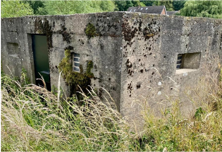
Figure 6. Pillbox converted to bat roost/ hibernacula opposite Walton south. Note the padlock cover to protect the padlock against vandals.
