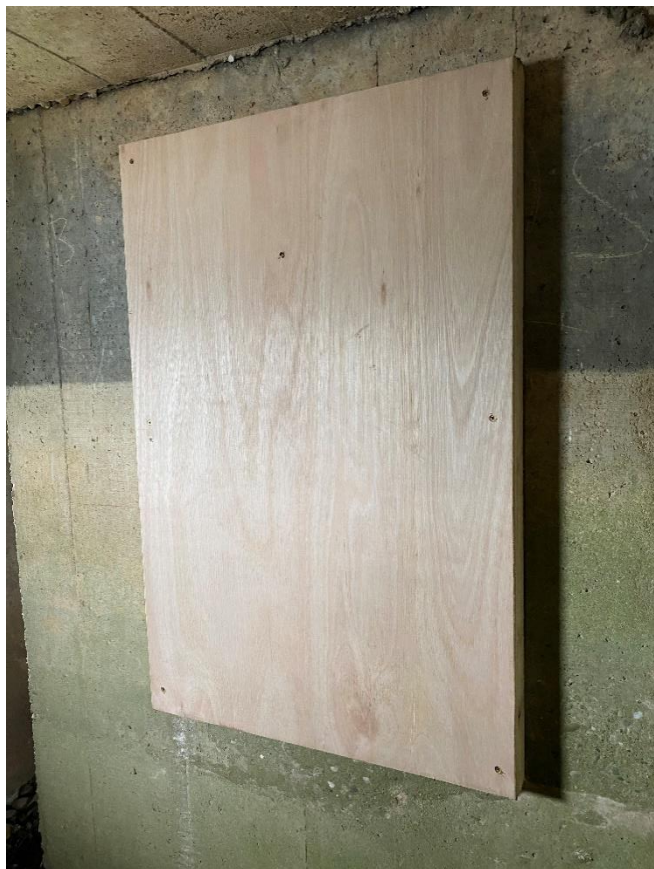
Figure 8. A plywood cover fitted to either side of the internal blast wall raised on 20mm deep batons at each side, allowing a narrow crawling space for the bats to roost or hibernate behind.
