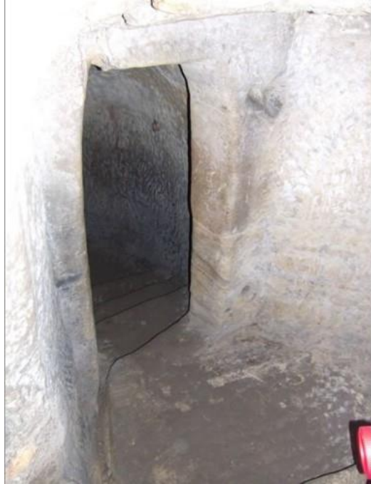
Doorway within Pontefract Hermitage
