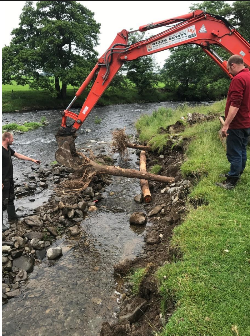
Figure 18. Photograph showing installation of Larch root bole flow deflectors.
