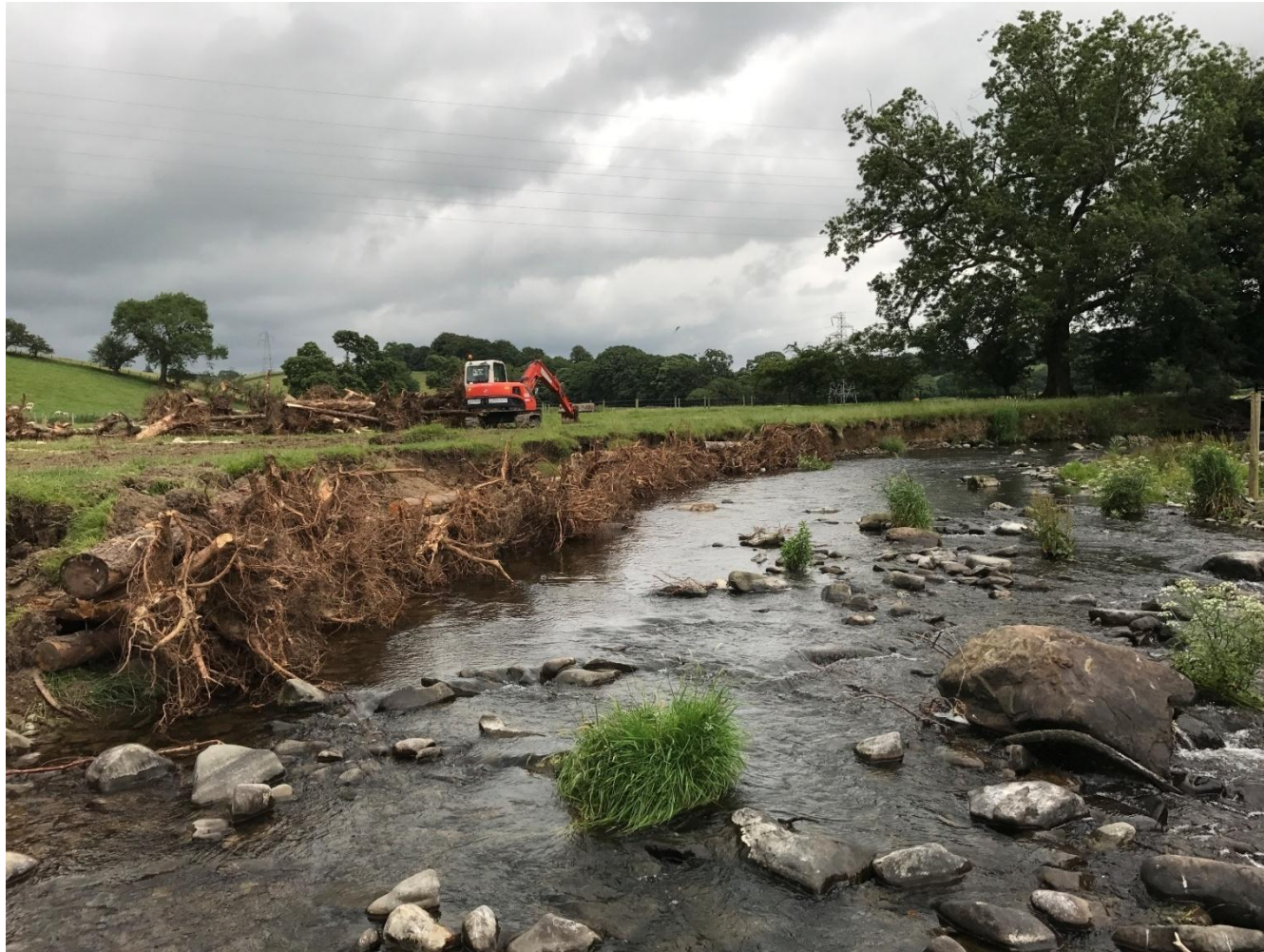
Figure 20. Photograph showing installation of Larch root bole flow deflectors.
