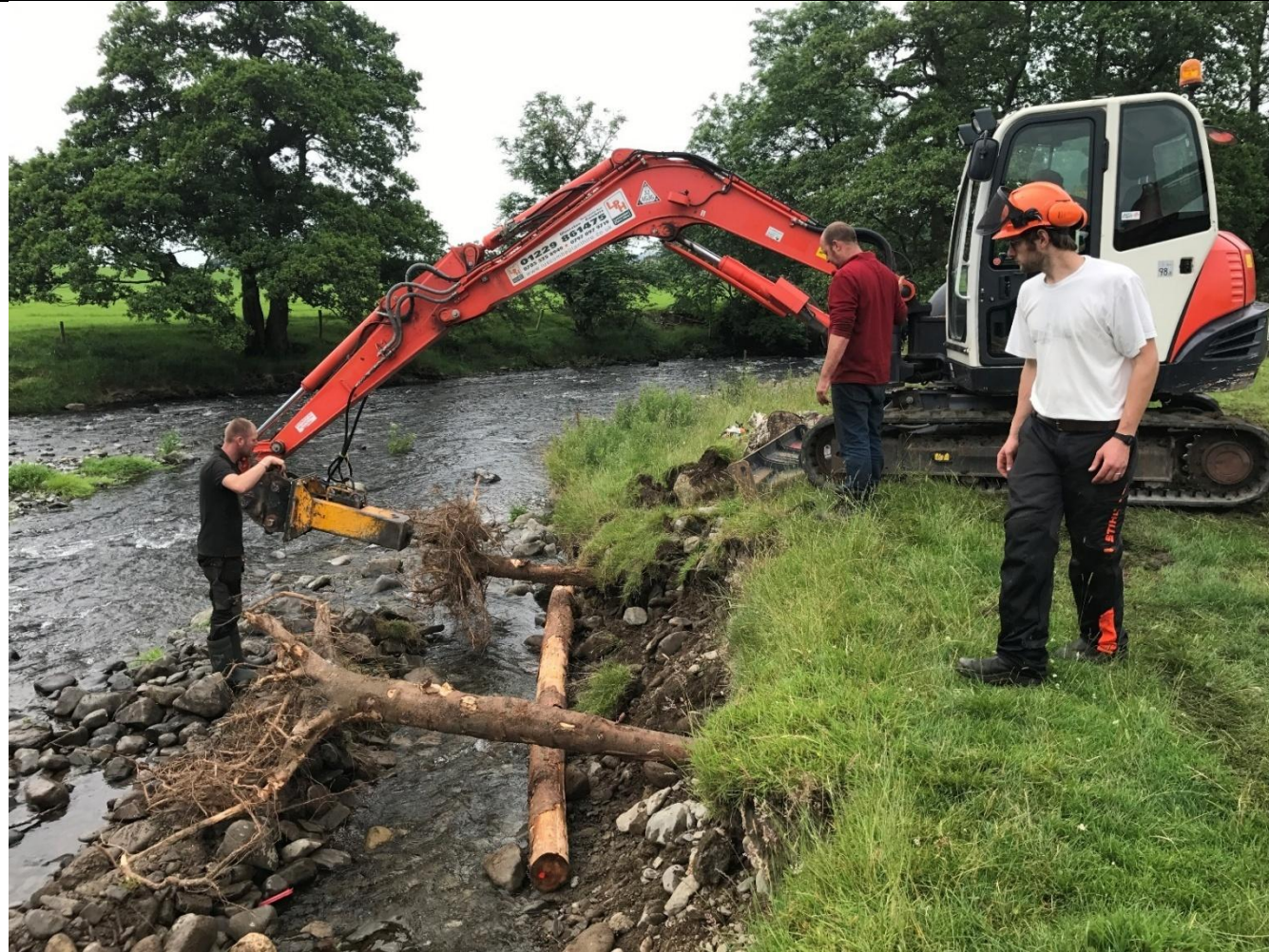
Figure 19. Photograph showing installation of Larch root bole flow deflectors.
